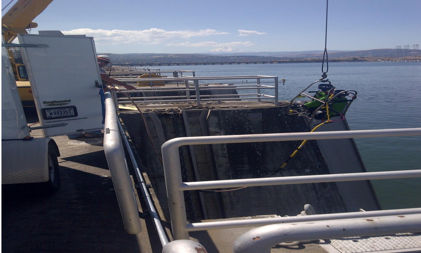
ROV deployment for sonar scan of turbine intake trashracks
